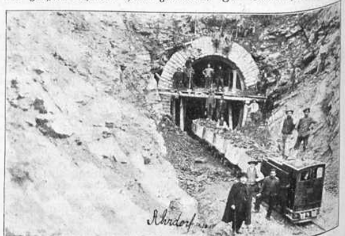
Ahrdorfer Tunnel (392 m lang).
